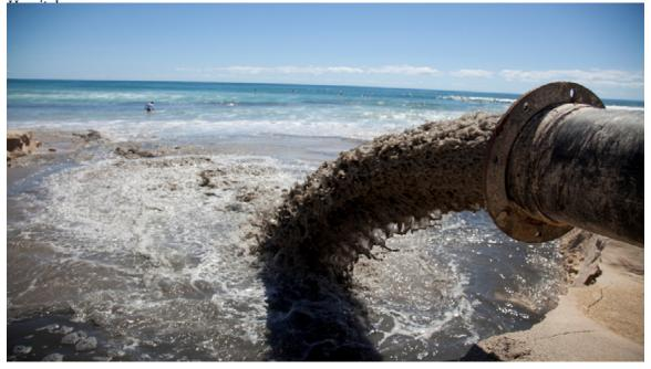
Figure 2: Combined sewer overflow. Image courtesy of Lineal.co.uk.
