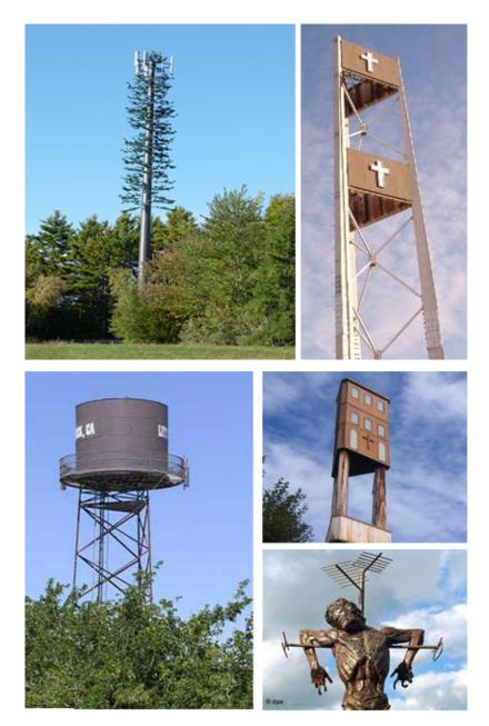
Figure 12. Cell phone towers concealed as trees, water towers, and church steeples. Images courtesy of Wikimedia.com, Weburbanist.com, Nationalgeographic.com, Paloaltofreepress.com.
