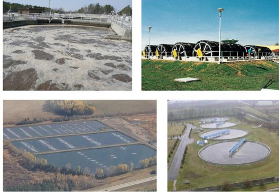
Figure 58: From top left to bottom right: activated sludge basin, rotating biological contactor, lagoon, settling tank. Images courtesy of Biostrainz.com, Rotatingbiologicalcontactor.com, Rockymtnhouse.com, Tankonyvtar.hu.
