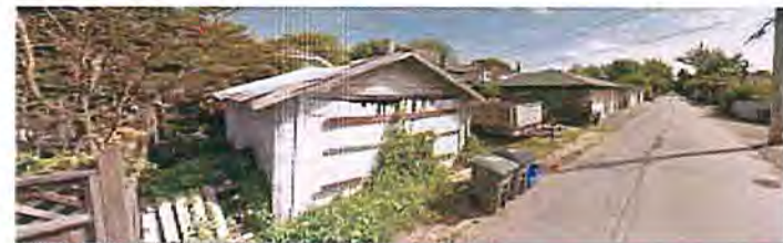
DETACHED HOMES FROM STREETSCAPE
