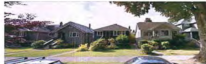
DETACHED HOMES FROM STREETSCAPE
