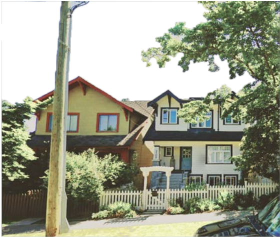
2104-2108 Maple Street (Google Earth, 2022)
