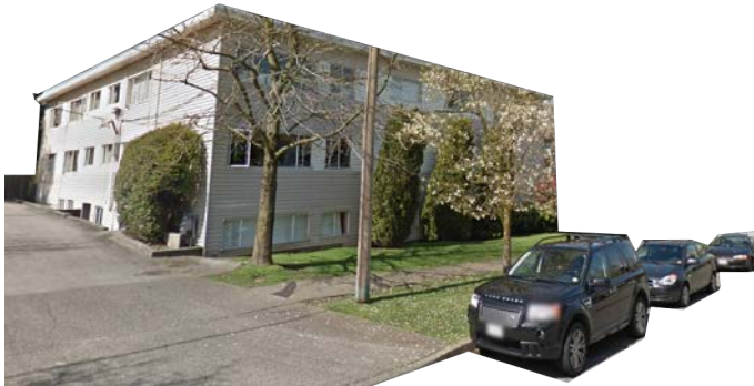
2014 Maple Street (Google Earth, 2022)
