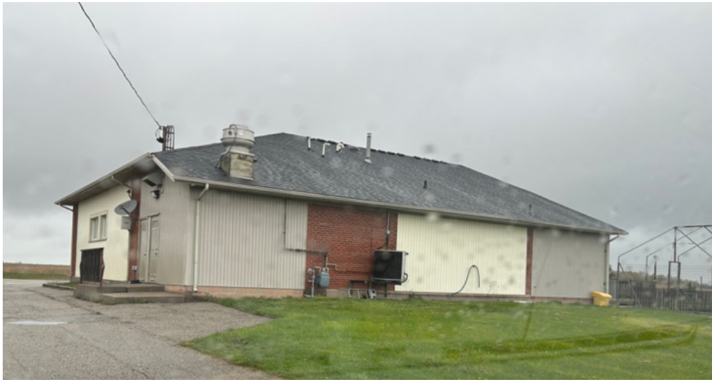
Figure 62 London & St. Thomas Croatian Cultural Centre, a windowless, gated community centre that faces its back towards the adjacent public street, 2024
