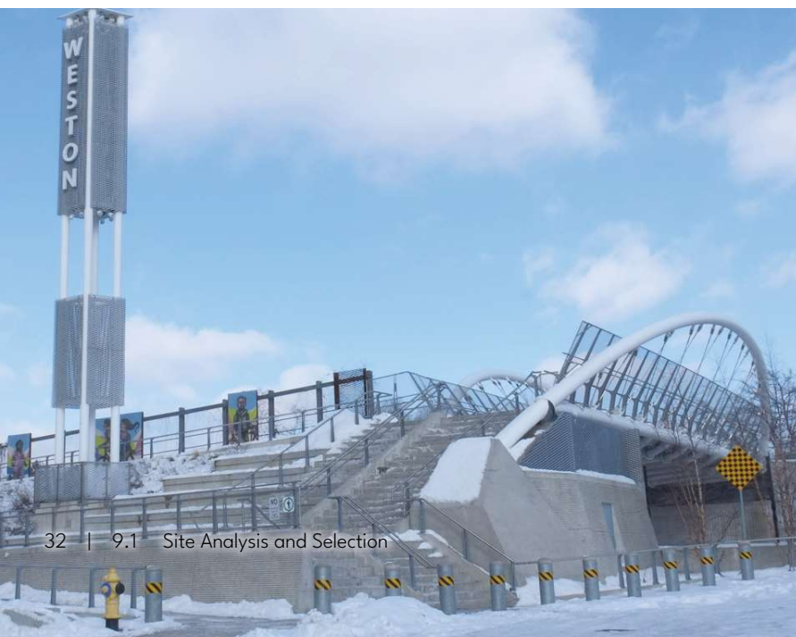
Figure 9.1.34.: New pedestrian bridge, stairs, and neighbourhood beacon 136
