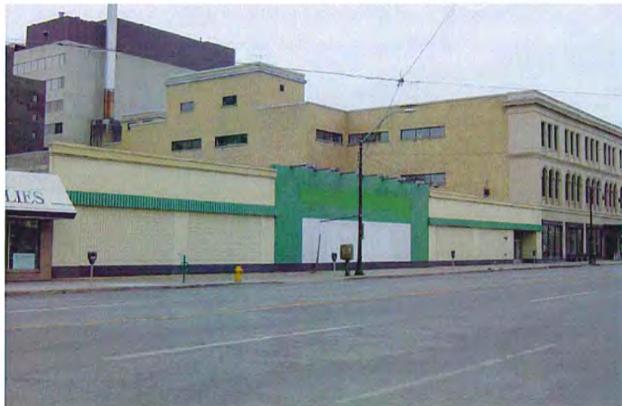
Figure #9- Photo from 3 rd Avenue Looking Southeast
