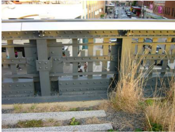
Refurbished iron railing
