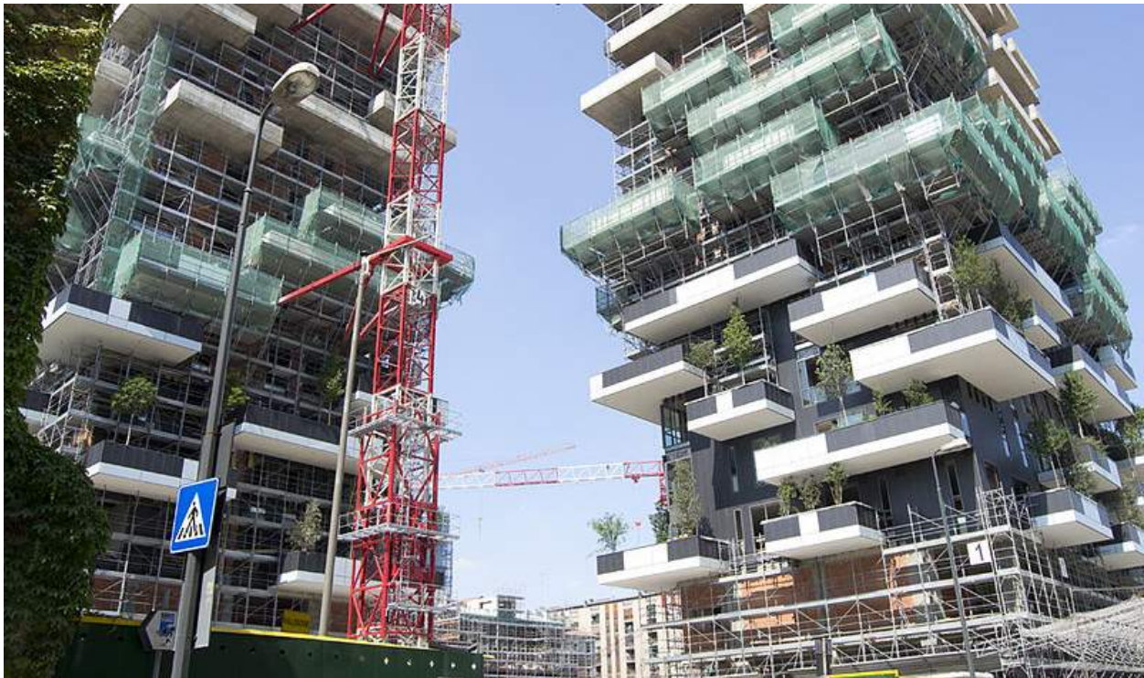
Bosco Vertical towers under construction
