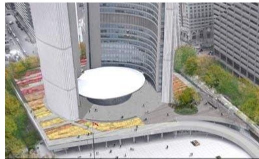
Aerial of the rooftop garden
